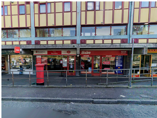
The block of flats and businesses beneath them, known as The Views, are due to be demolished to make way for a new development. Image: Google Maps
